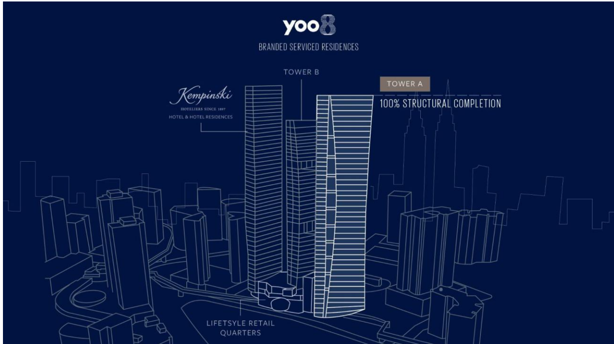
PIC 002: Located at the heart of the Golden Triangle of KL City Centre, 8 Conlay's twin residential towers - YOO8 serviced by Kempinski, now celebrates the structural completion of Tower A and onward to its handover by end of 2022.
