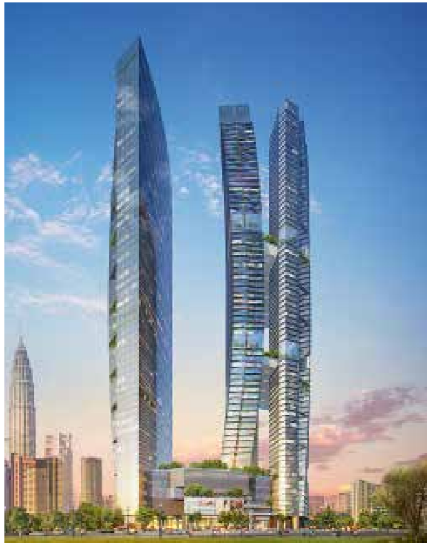
8 Conlay will be the world's tallest twisted twin residential towers upon completion.
